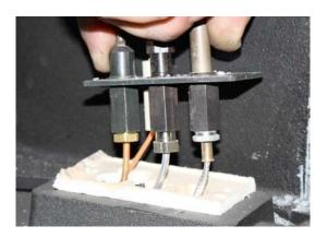
9. Remove the old gasket material from under the pilot assembly and discard.
