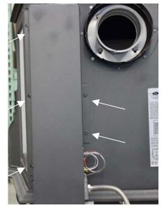
11. Lift the cover upward away from the knobs and disconnect the wire from the underside of the piezo igniter. The on/off switch may remain connected.
